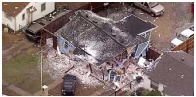
**Figure 1**: 3534 Espanola Drive shown. The home was blown from its beams, slightly rotated destroying virtually every internal structure and mechanical system in the home.
